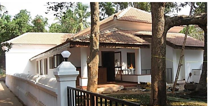
The Contemporised traditional building with arrested decay and the addition of new design elements (Source: Author)
