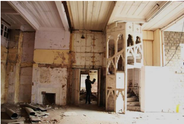
Shimla Town Hall interior spaces before conservation
